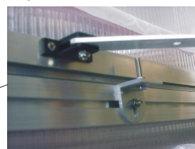
Window fixing with screw 4,2x16 to screw down
